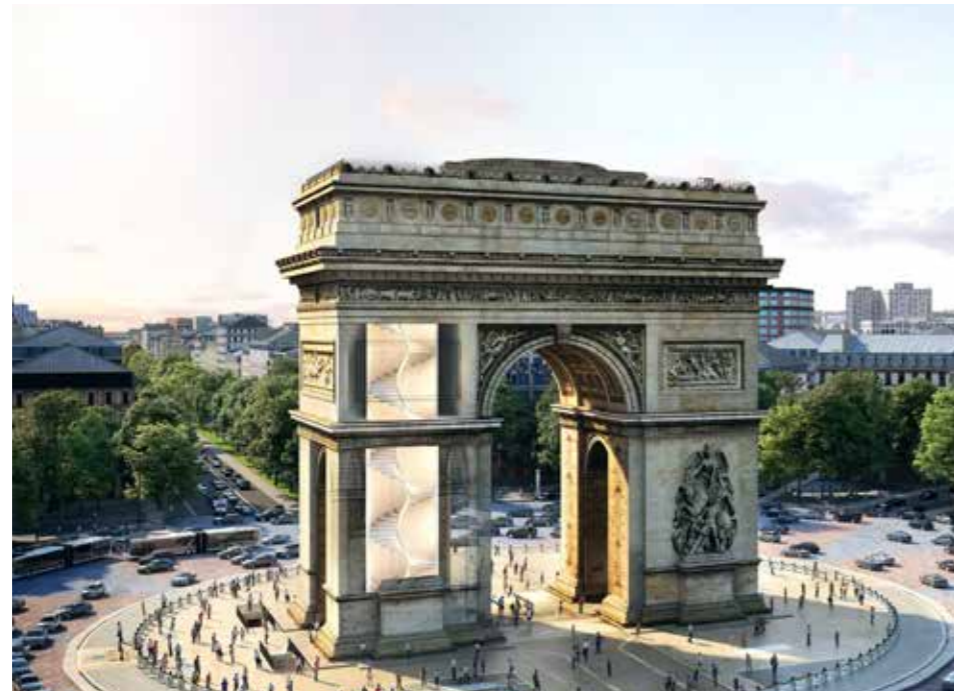
Arc de Triomphe, Paris - Stairs in UHPC
